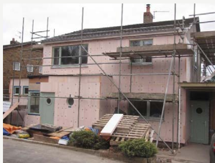
Figure CS1.1 Front elevation prior to render or cladding
