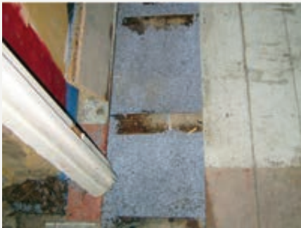
Figure CS8.3 Void filled with insulating beads
