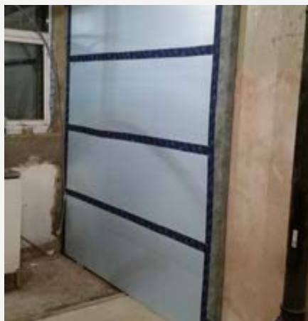
Figure CS5.3 Internal wall insulation on party wall exposed to the outside
