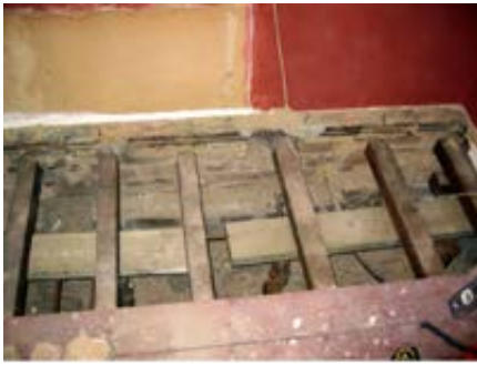
Figure 4.15 Shaftesbury Park: pre-retrofit ground floor and joists
