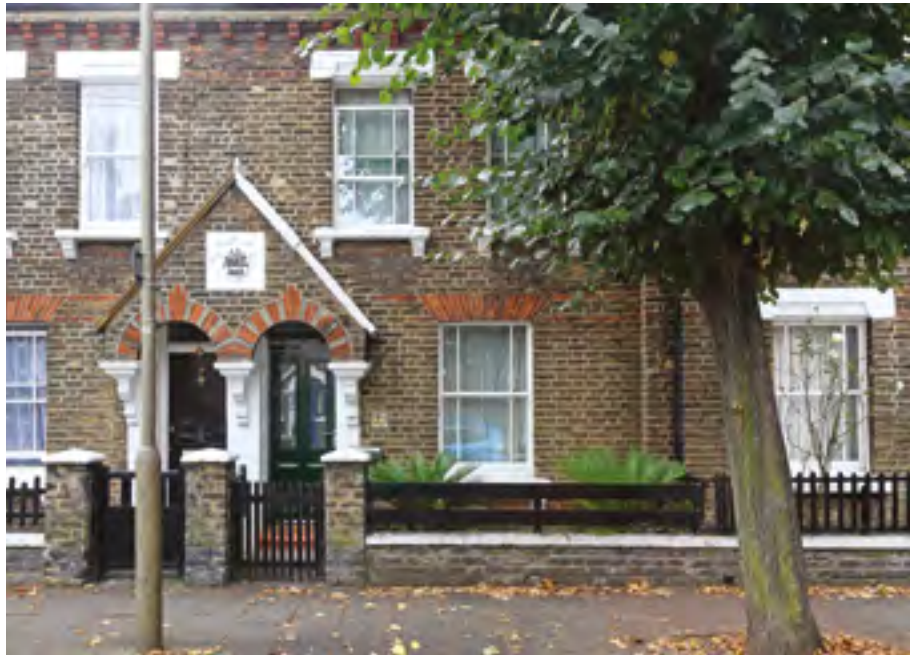
One-off property retrofit
