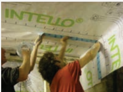
Figure CS3.1 Installation of air/vapour barrier during original retrofit
