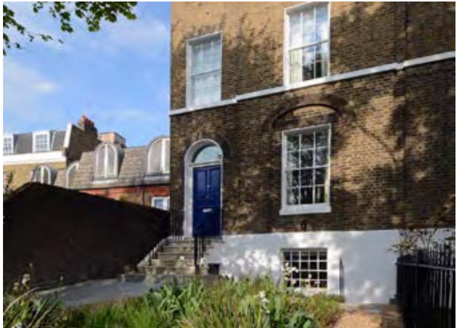
One-off retrofit. Completed October 2013.
