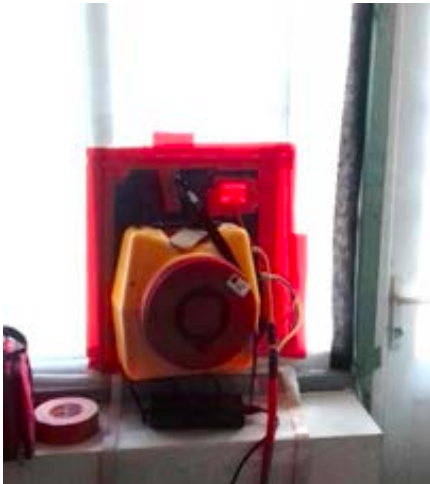
Figure CS5.1 Blower door test through window in 2015
