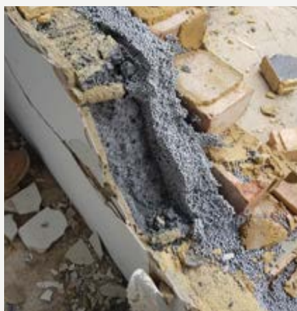
Figure CS5.5 Step 1: cavity wall insulated with polystyrene beads being removed
