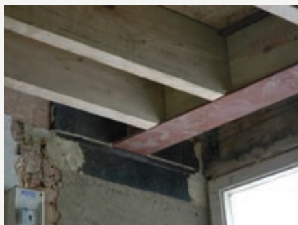
Figure CS7.1 Joists re-hung on steel beam set in party walls
