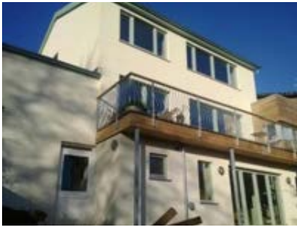
Figure CS1.7 Rear elevation with external wall insulation and balcony
