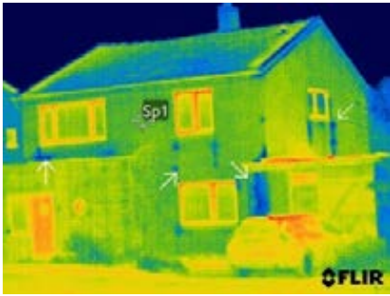
Figure 4.13 Blaise Castle: infrared image of front (west) and side (south) elevations (arrows indicate surface condensation with run-off from aluminium sills and interface with car port roof; this finding is subject to further investigations to confirm the cause)
