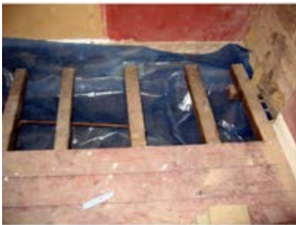
Figure 4.16 Shaftesbury Park: ground floor membrane below joists
